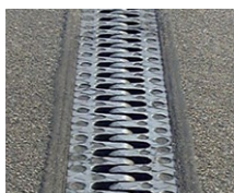
Cantilever finger joints
