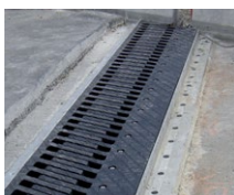
Sliding finger joints
