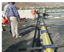
Fanja Bridge (Oman)
