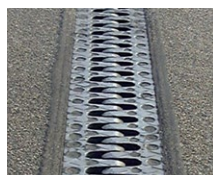
Cantilever finger joints
