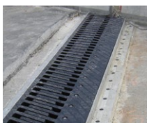
Sliding finger joints
