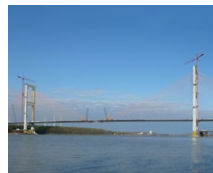
Audubon Bridge (USA)
