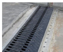
Sliding finger joints
