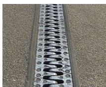
Cantilever finger joint
