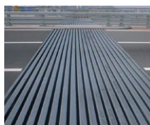
Modular expansion joints
