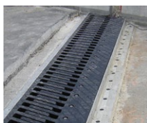
Sliding finger joints
